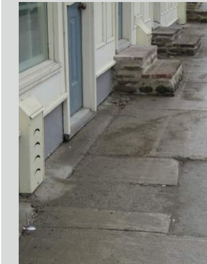
Business entrances not level with sidewalk- requires stairs up into buildings. Ramps without handrails provide obvious challenges and add to obstruction on street.
