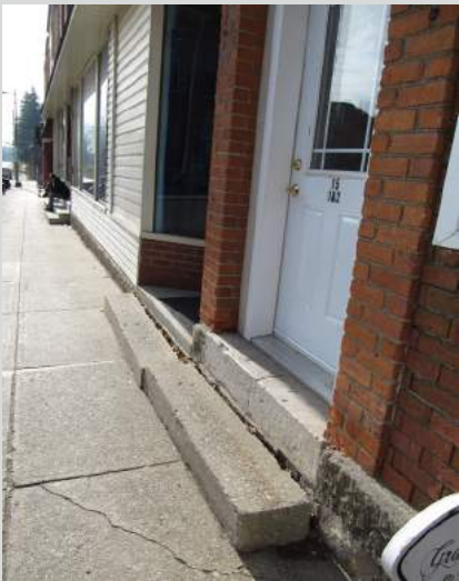
Business entrances not level with sidewalk- requires stairs up into buildings. Ramps without handrails provide obvious challenges and add to obstruction on street.
