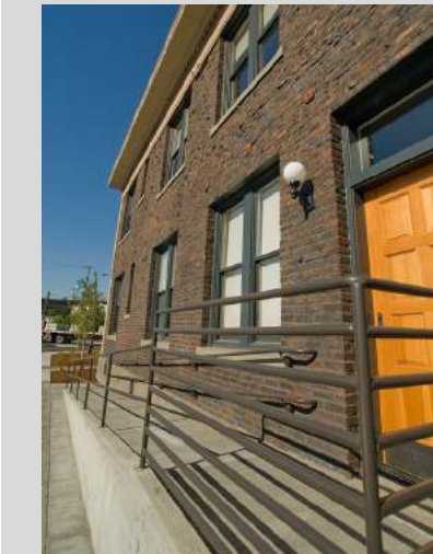
Concrete ramp with guardrail provides access to historic building. Note colour of handrail.
