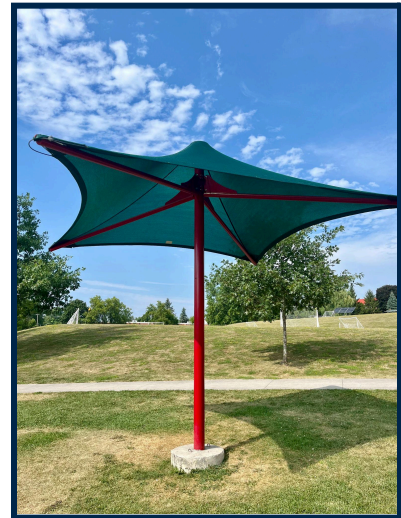
Figure 3.2: Shade Structure at Kennedy Park
