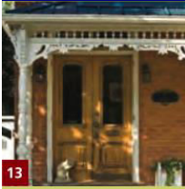
7 Centre Street Hipped Roof
