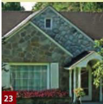
94 Old Hastings Road Cobblestone Chimney
