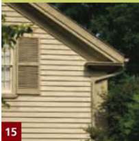
12 George Street Enhanced Fascia
