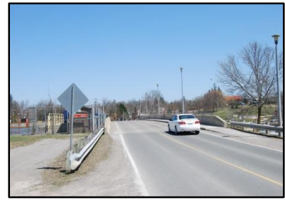
3. Two Lane Municipal Bridge over Trent-Severn Waterway Control Structure
